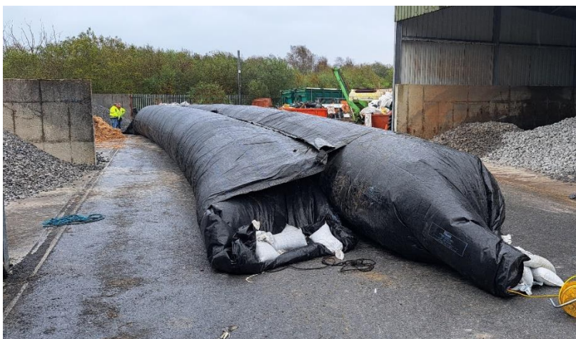
BALLINASLOE FLOOD DEFENCE AQUADAM TESTING
