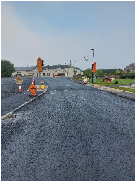
OVERLAY WORKS COMPLETED IN R332 BARNADEARG
