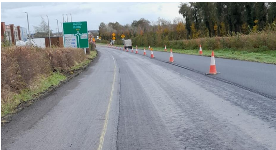
R446 DUAL CARRIAGEWAY WORKS - COMPLETE
