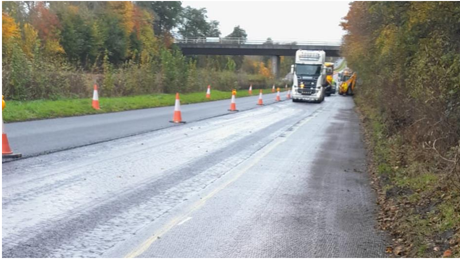
R446 DUAL CARRIAGEWAY WORKS - COMPLETE
