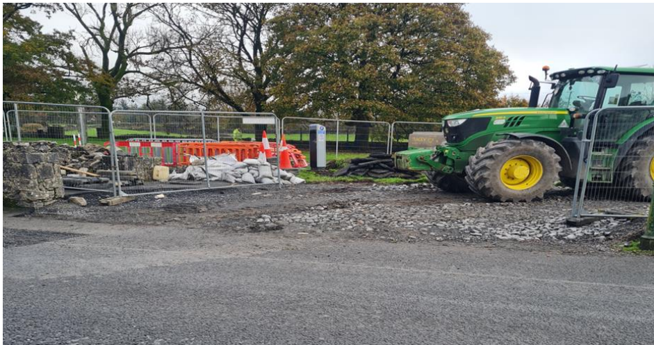
ATHENRY NETWORK UPGRADE ONGOING
