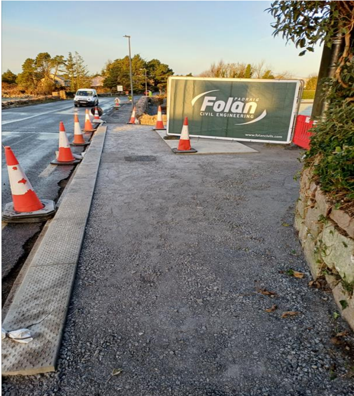
BUS SHELTER IN CASLA, UNDER CONSTRUCTION
