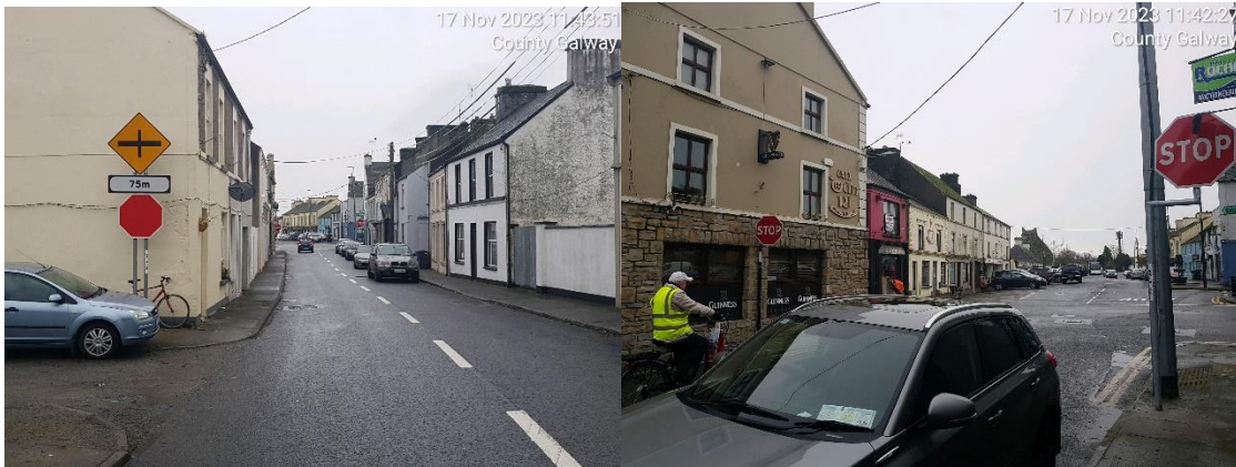
UPGRADE TO SIGNAGE ON CASTLE STREET DUNMORE APPROACHING TOWN CENTRE JUNCTION
