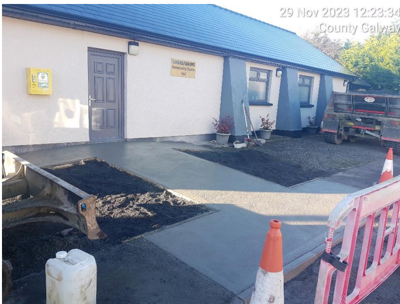
FOOTPATH REPAIRS WORKS TO ENABLE DISABLED ACCESS TO GARRAFRAUNS COMMUNITY CENTER
